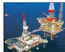
Operational safety on offshore platform
